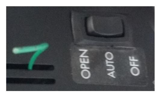
The handicapped accessible doors should **ONLY** be propped open by toggling the switch on the mechanisms to "**OPEN.**" Putting objects in front of these doors runs the risk of burning out the motor.
